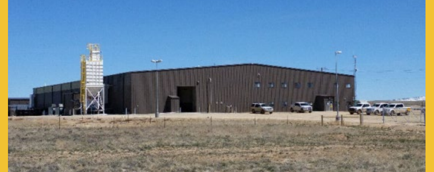
UR-ENERGY'S OPERATING LOST CREEK ISR PLANT
